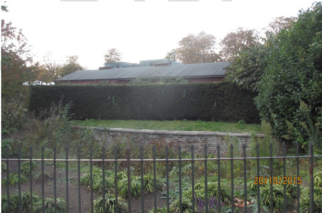
Photograph 2: Existing stable building to be demolished and its relationship with the Bastion Wall (from Western Carriage Drive)
