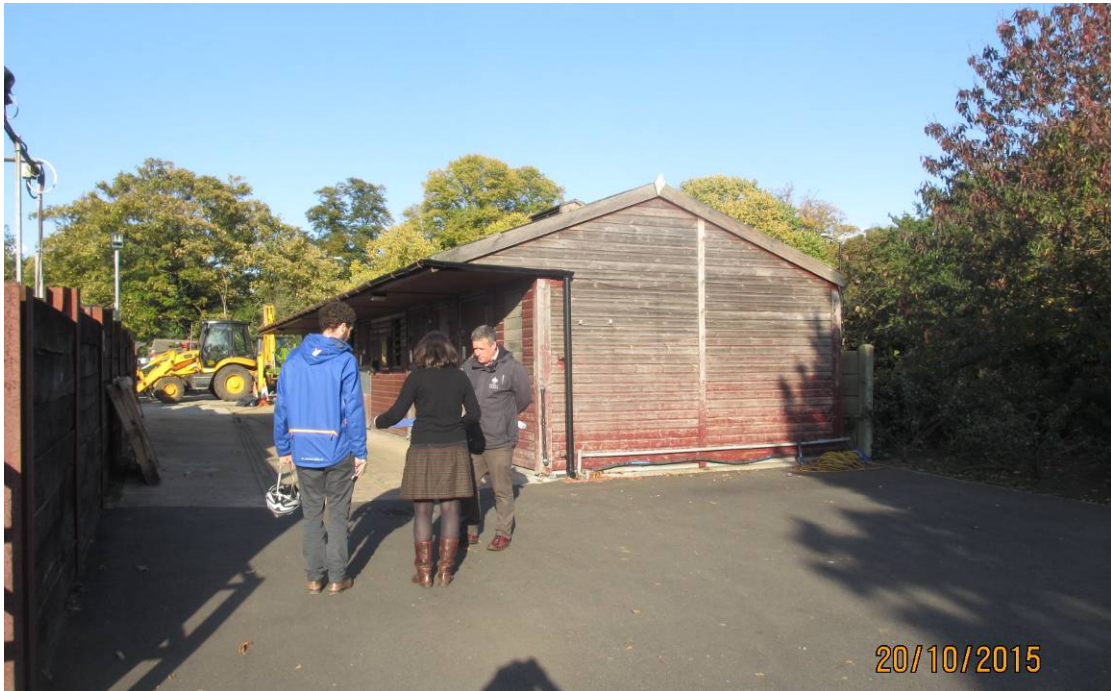
Photograph 1 (above): Existing stable building to be demolished (from within site)
